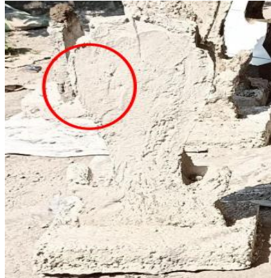
Gambar 1. Defect batu nisan
