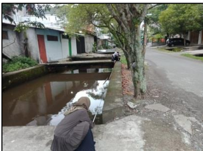
Gambar 5. Pengukuran Drainase Eksisting
