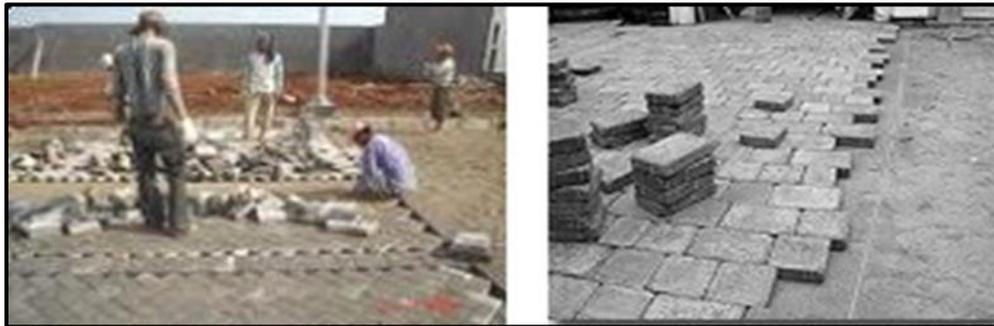
**Gambar 5.** Pemasangan concrete paving block
