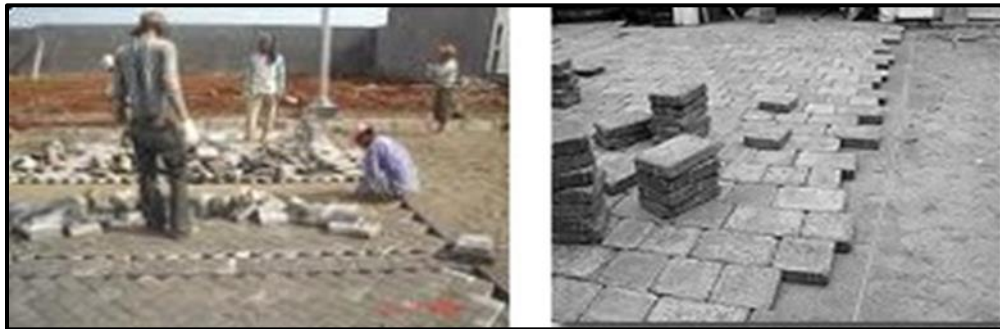
Gambar 5. Pemasangan concrete paving block
